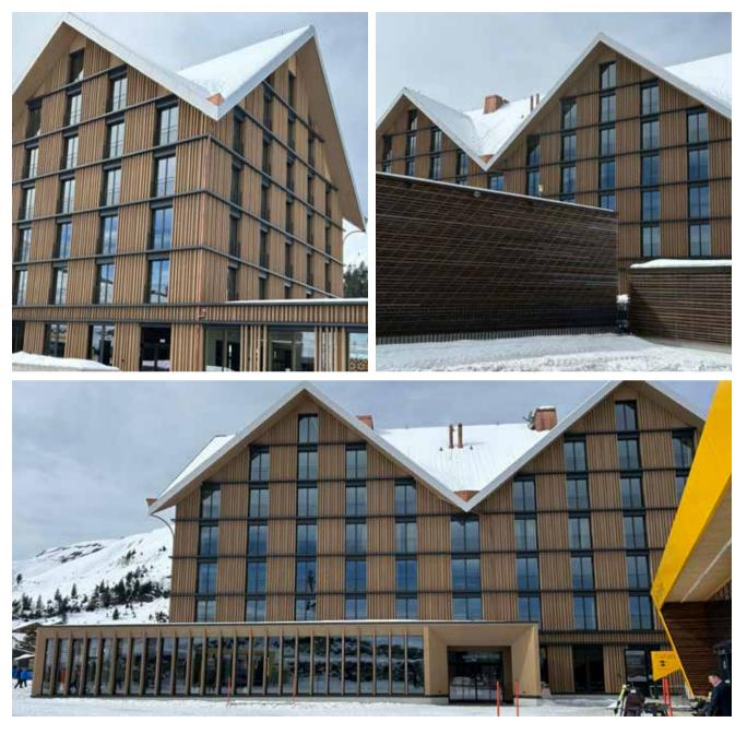
The Hotel Stoos Lodge is located at 1 300 metres above the sea level and stands in the middle of a ski resort in the canton of Schwyz. To renew the façade, a total of 4 600 m<sup>2</sup> wood was treated with Sunprimer HWP and Hybrid Wood Protector.
